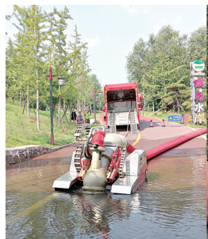
“龙吸水”抽排涵洞积水
